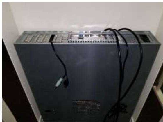
Speaker cable extracted and Monitor Cables routed over the computer
